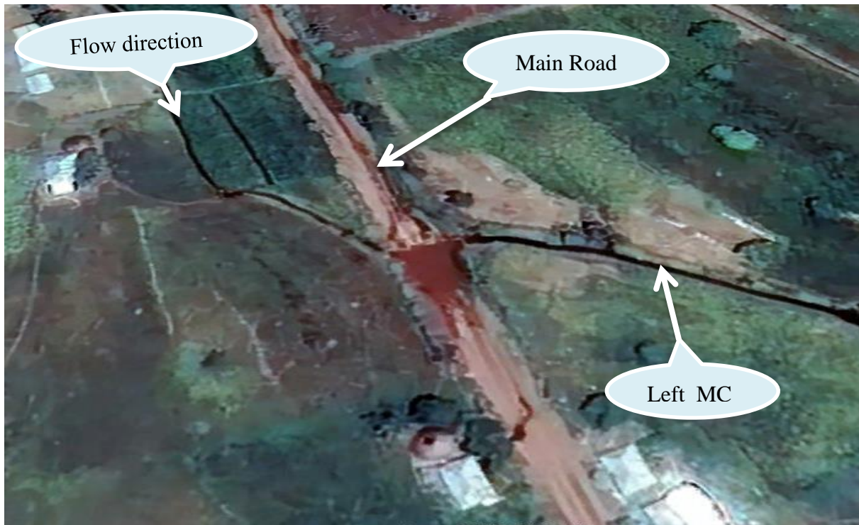
Figure 2 Condition of left side main canal
