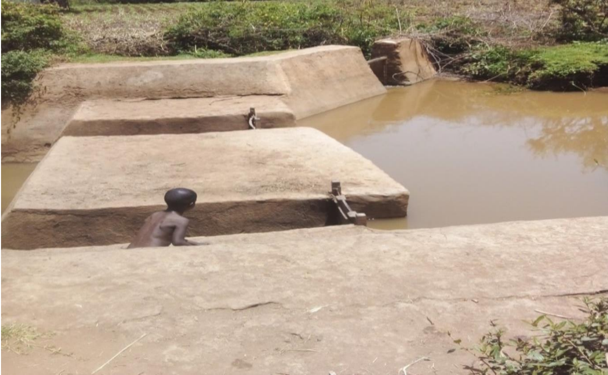
Figure 6 Headwork of Hargaya irrigation scheme
